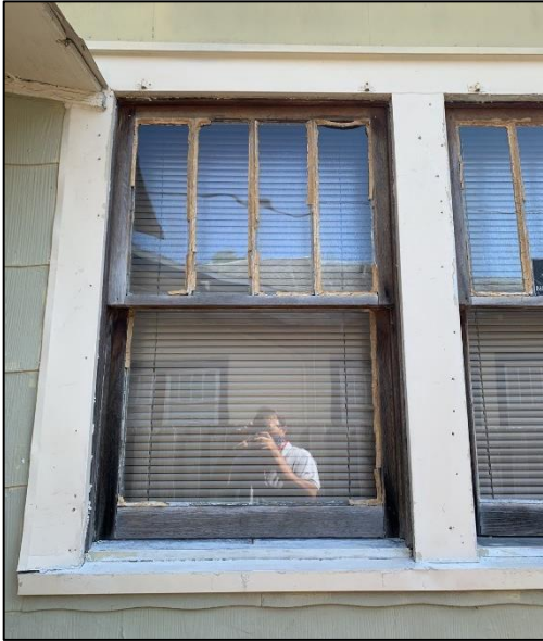
Figure 2: Existing wood windows
