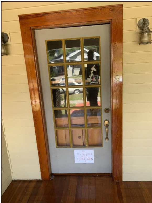
Figure 4: Existing front door
